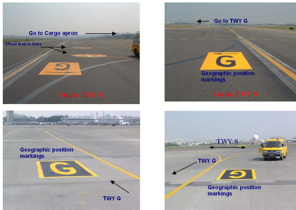
FIGURE 4d After completion of marking improvements at the intersection of TWY S, G and entrance to cargo apron
