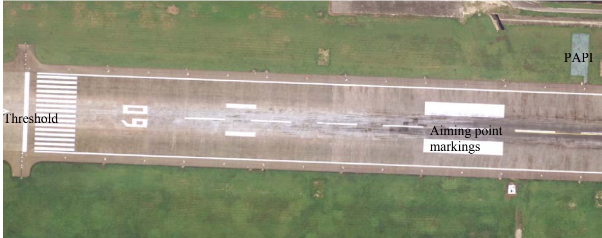
FIGURE 2a Geometric relationship between aiming point markings and the PAPI on the 09 runway direction at KHH
