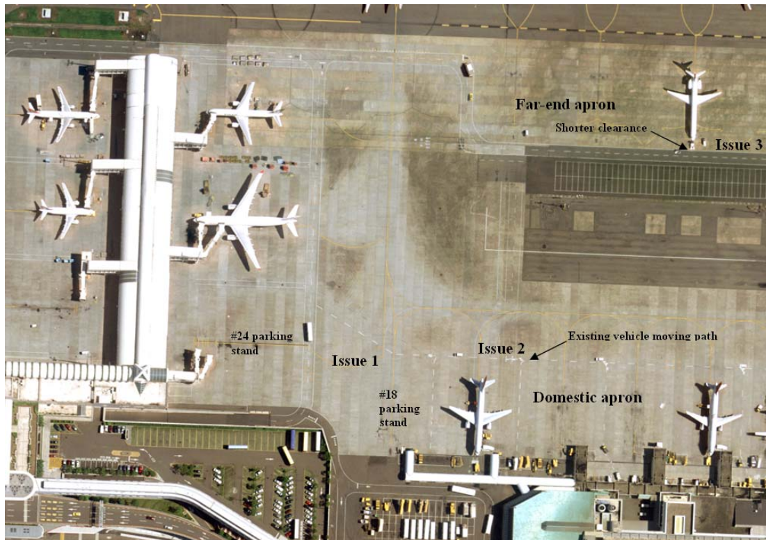
FIGURE 6a Identified issues in the far-end apron and domestic aprons
